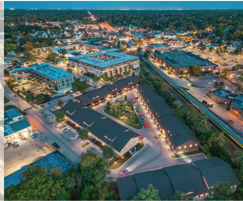
Currently Under Construction (Mylo Development)
